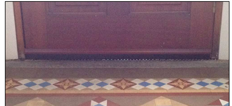
Draught-proofing strips can be easily applied to interior side of external door
